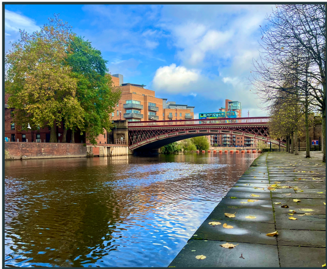
Leeds, Crown Point Bridge
